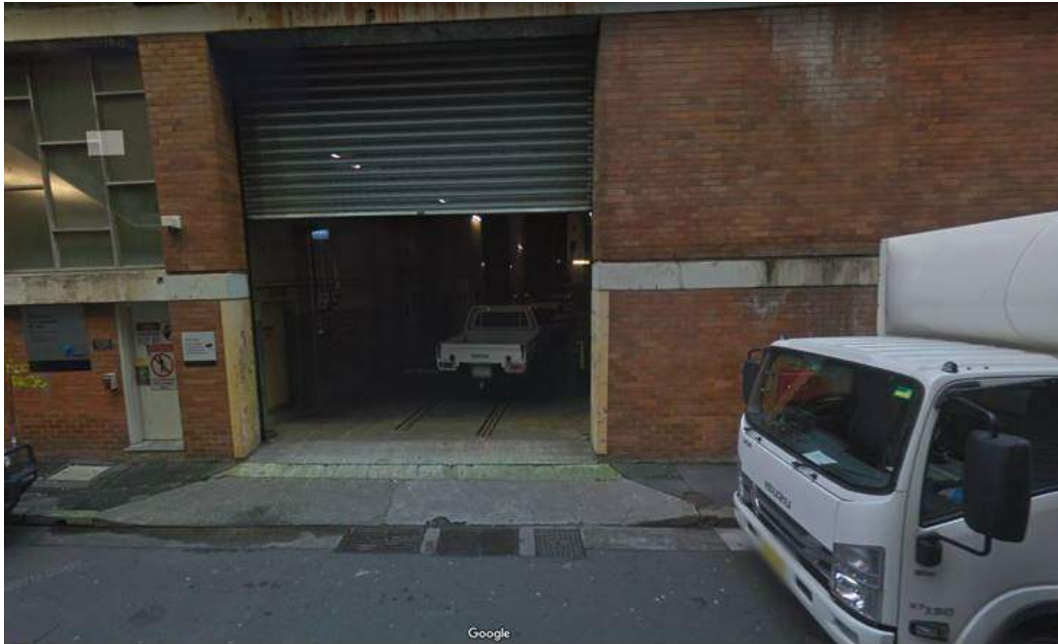
Figure 19 - Existing Ausgrid vehicular entry
