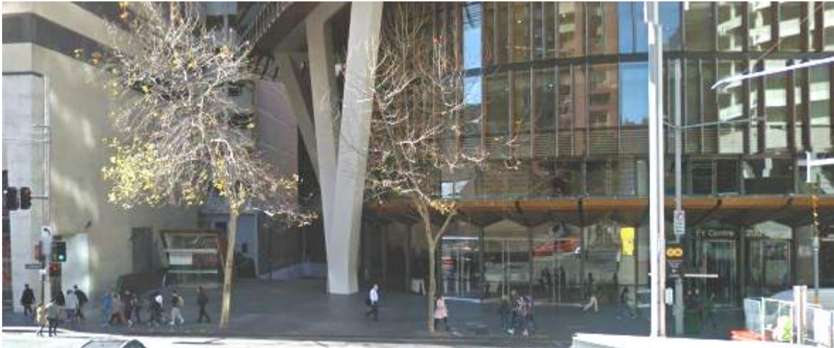
Figure 4 200 George Street and Crane Lane
